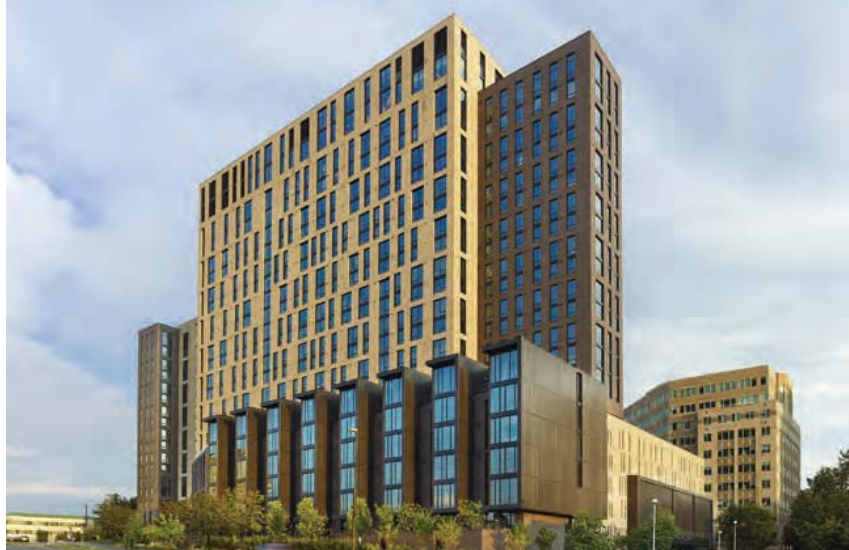
The Signature at Reston Town Center, Reston, VA
